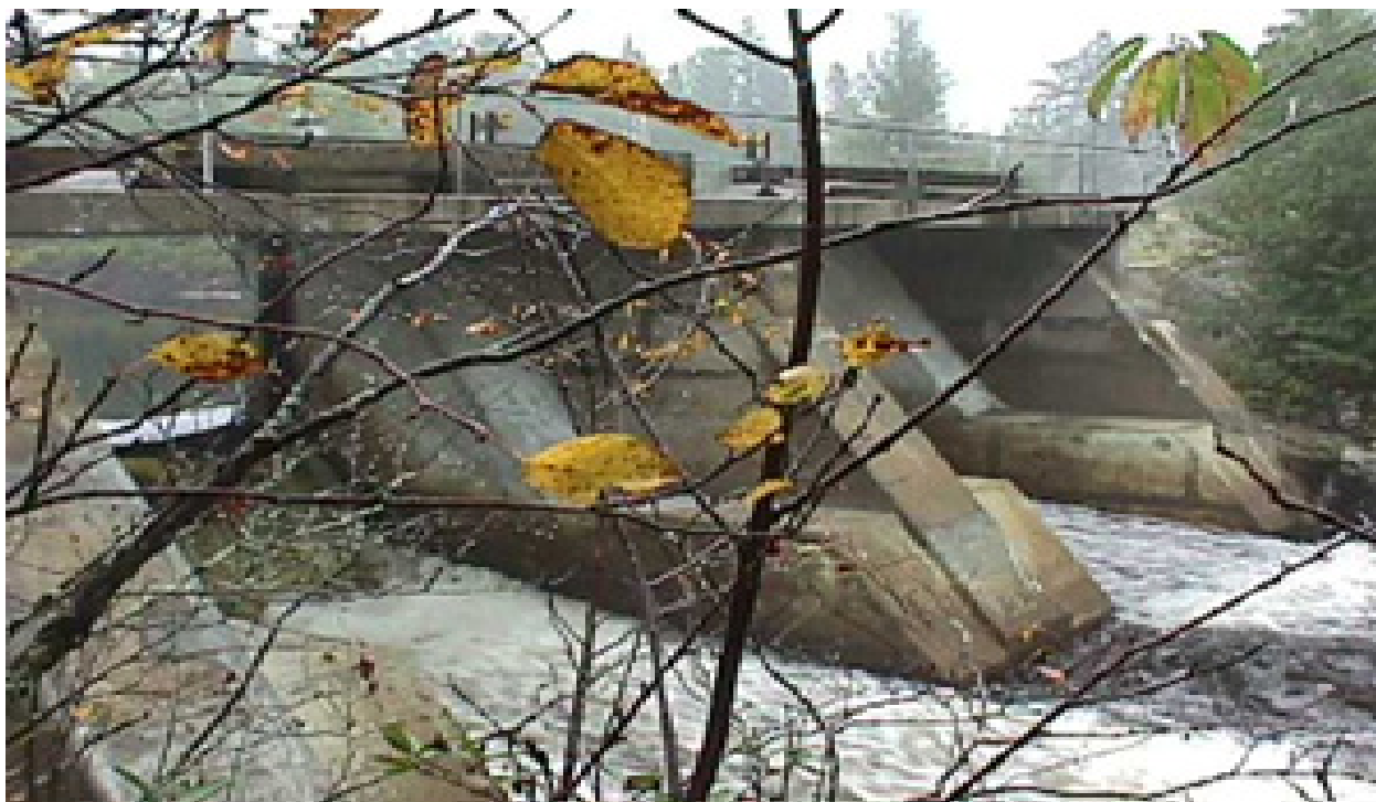
Figure 2: Barrage Giroux, source CEHQ
